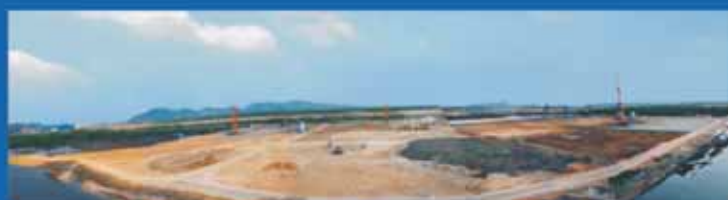
SP-PSA Construction Progress – February 2008
